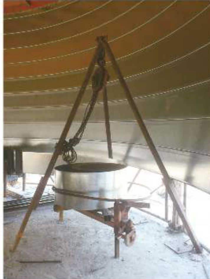
2. Decoiling steel plate
