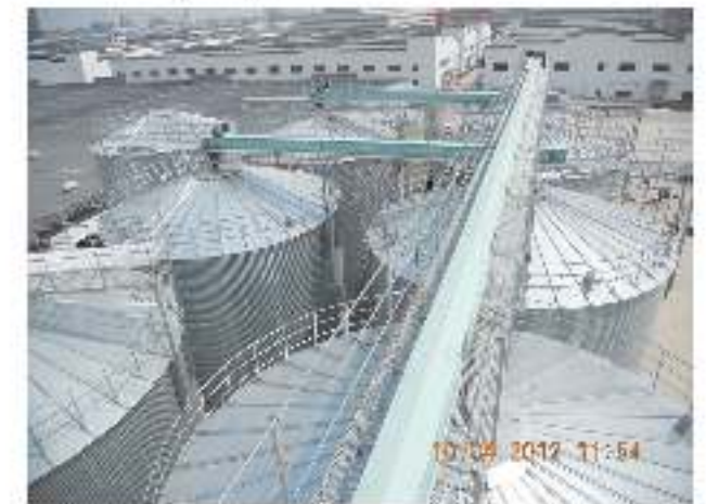
Grain Transportation--Belt Conveyor
