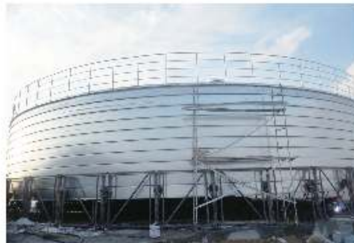
5. Coiling steel plate
