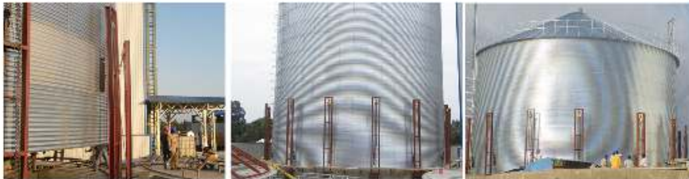
2. Silo body installation
