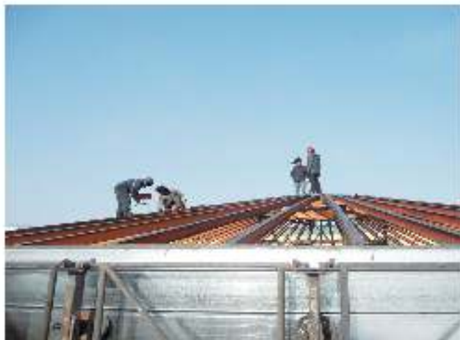
4. Silo roof welding
