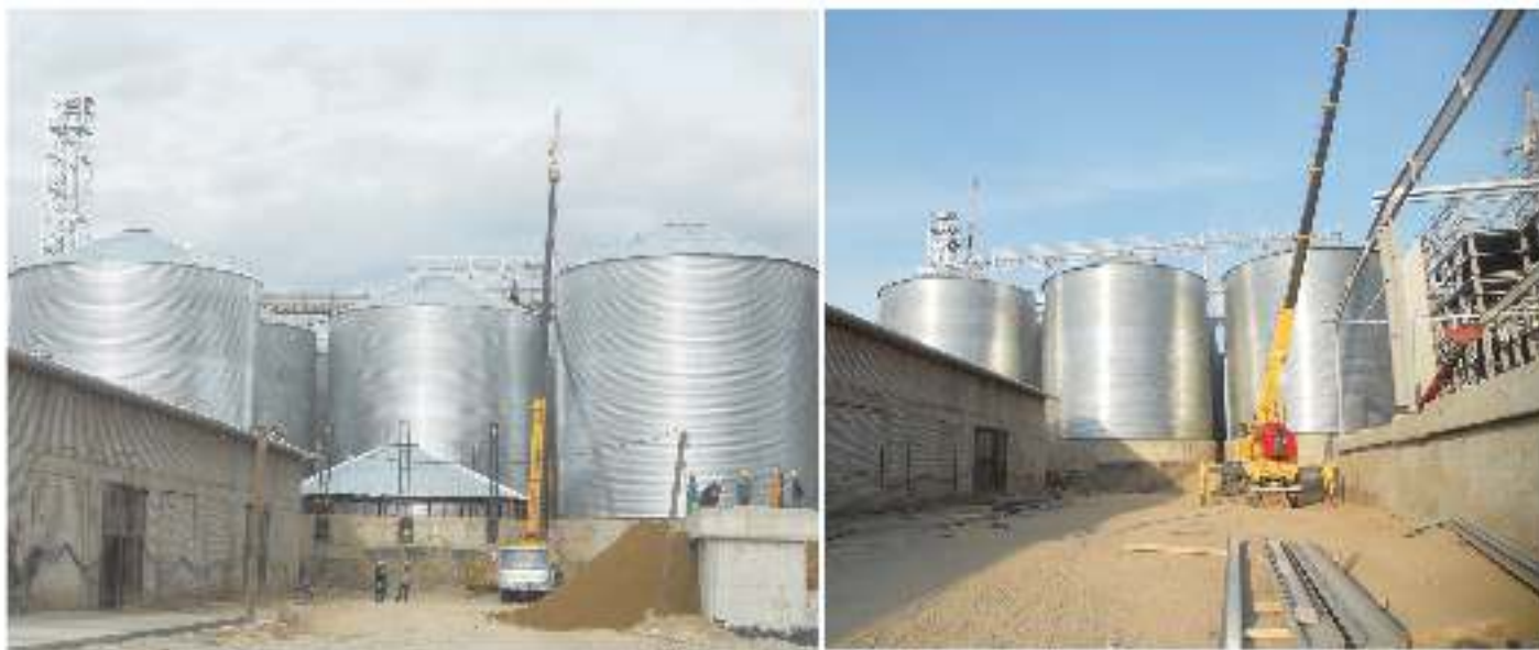
3. Silo installation finish
