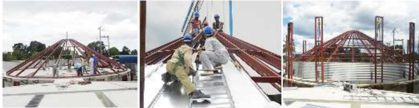
1. Silo roof installation
