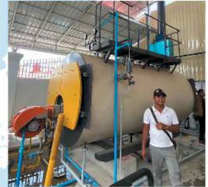
8 Ton Gas Steam Boiler In Philippines
