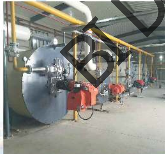
3 Ton Oil/Gas Steam Boiler In Peru
