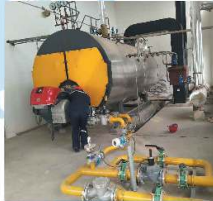
10 Ton Oil/Gas Steam Boiler In Iran
