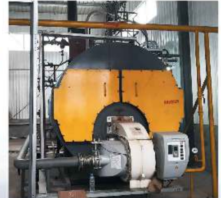
1 Ton Oil/Gas Fired Steam Boiler In Ecuador
